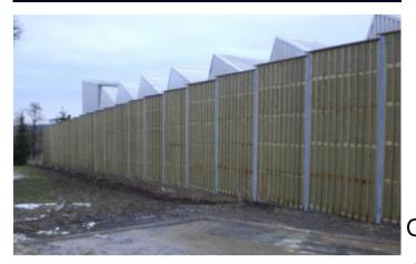
Modular or basic building block design that enables you to meet your specific noise abatement requirements without the cost of custom designing. - Fixed or Mobil solutions -
